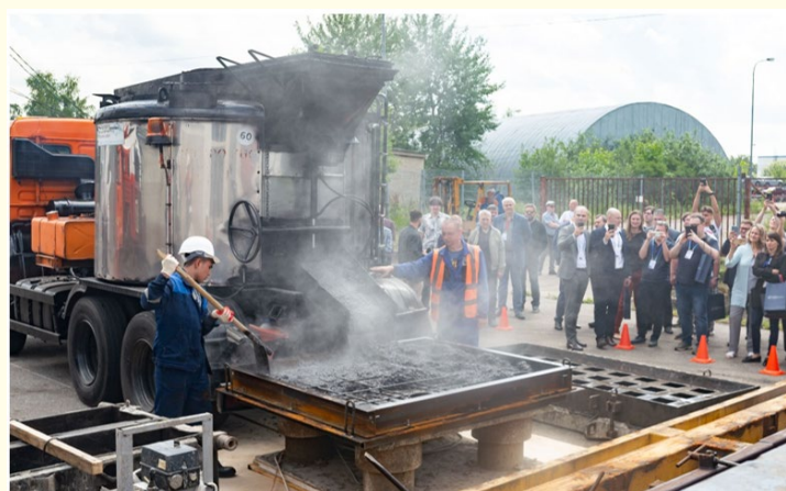
Figure 5: The section of forming of sulfur concrete road slabs in MADI.
