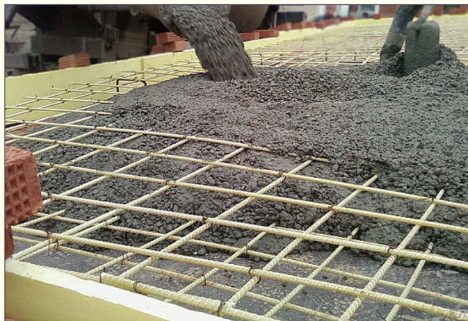
Figure 11: Reinforcement with composite reinforcement during the manufacture of road slabs.
