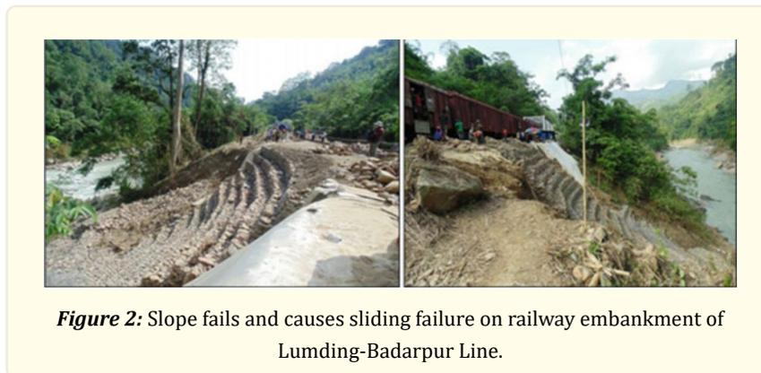
**Figure 2:** Slope fails and causes sliding failure on railway embankment of Lumding-Badarpur Line.
